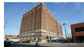
Sterling Bay purchases 1000 W Fulton, a 10-story 385,000 SF windowless cold-storage building constructed in 1920
